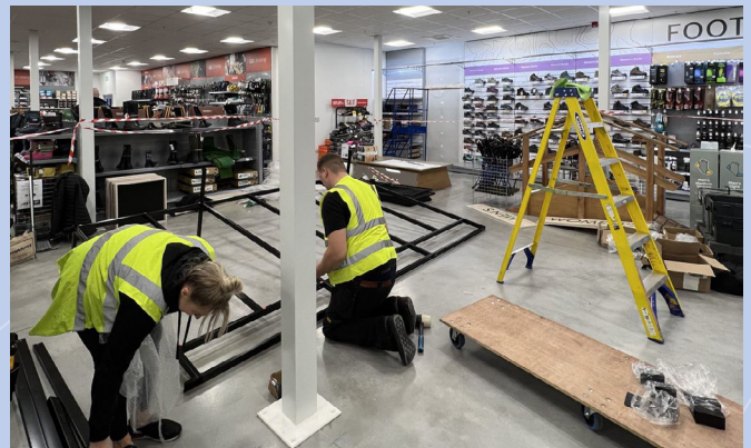
The racks installation site.
